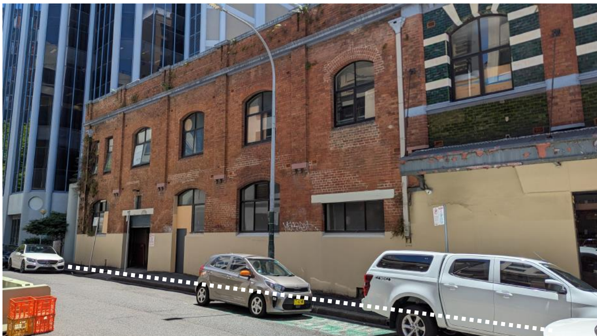
Figure 3: Site viewed from Valentine Street
