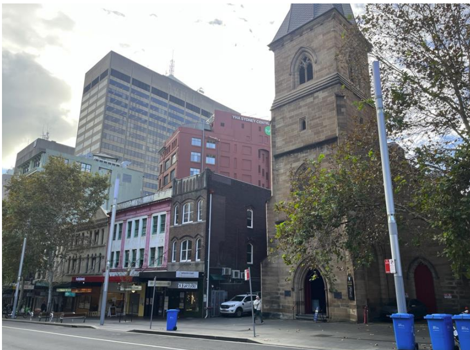
Figure 10: Looking east from subject site
